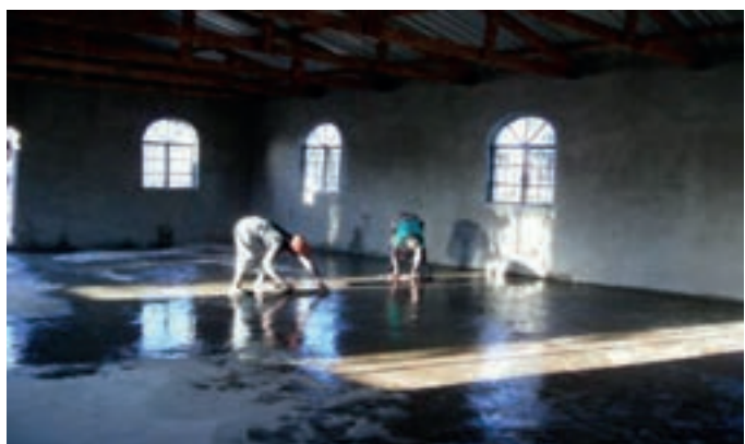
Polishing the cement floor
