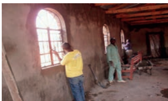
Fitting window frames
