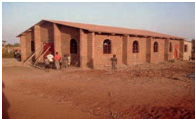
The new hall at Lilongwe
