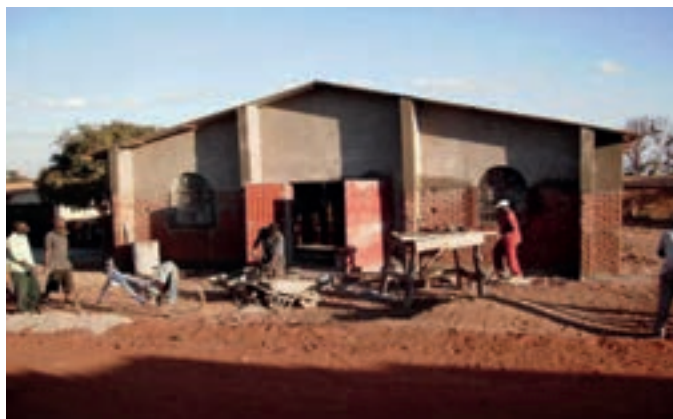
Plastering the walls
