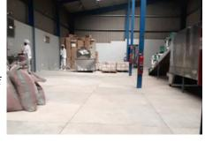
the concrete floor began cracking and dust was circulating with potential for contaminating the food. The new polished surface is easy to clean, and any liquid spillage will not stain the surface.
