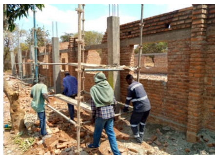
Building the pillars for the roof
