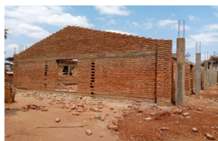
Pillars and ring-beam in place
