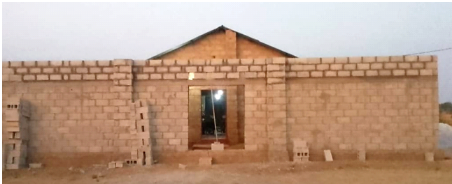
Construction has progressed steadily at roof level
